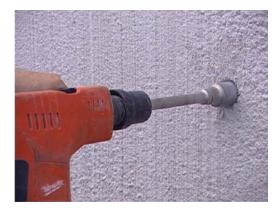
2. Use a masonry hole saw or a hammer drill with a small bit (to drill a series of holes around the perimeter of the hole). With a hammer and chisel start to work the area inside the small holes until the hole is the required size and shape.
