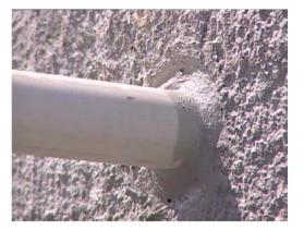
NOTE: Space the hole to avoid the concrete studs in the Superior Walls panel. Code Official may require a 'relieving arch' around the pipe. Seal carefully around pipe - standard wall warranty does not cover leaks around pipes.
