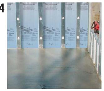
Pour concrete up to the screed board or back into the stud bays at the required finished slab height.
