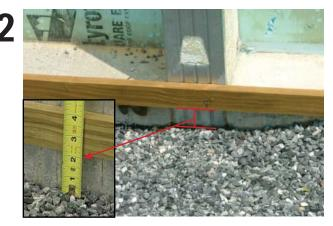
Fasten a piece of lath at the desired height of the concrete floor to form a screed board, or the screed board may be omitted to allow the concrete floor pour to flow between the stud cavities on top of the Superior Walls footer beam. Typically allow a minimum of 2" direct contact between footer beam and floor slab.
