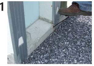
Bend slab connectors into concrete floor pour if provided.
