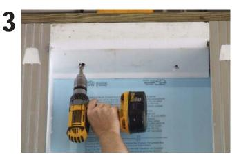
Using the holes provided in the concrete Bond Beam, drill through the sill plate from below.
