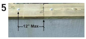
Sill Plate must be bolted within 12 inches of the end of all plate sections.
