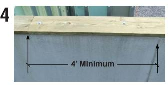
Sill Plate splice must be at least 4 feet away from foundation panel joint.
