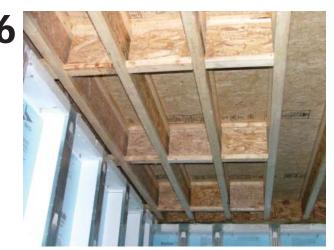
Install blocking and bracing between joists according to the instructions of the Builder Guideline Booklet.
