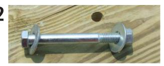
Bolt the Sill Plate with minimum 1/2" x 5-1/2" bolts with washers using the precast holes provided in the top Bond Beam.
