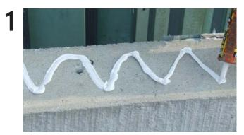
Construction adhesive is recommended between the Bond Beam and the Sill Plate (a 2x10 Sill Plate is recommended).
